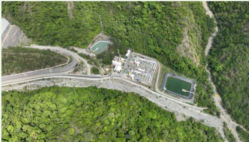
Water treatment plant of Continental Gold
