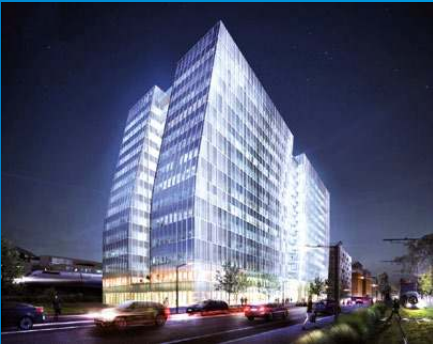
Skyscraper renovation 📍 Lyon, France Renovating a high-rise poses unique challenges, especially on upper floors. In Lyon, Ytong blocks provided an ideal lightweight, insulating solution for transforming the 14th floor, demonstrating their versatility in complex urban construction.
