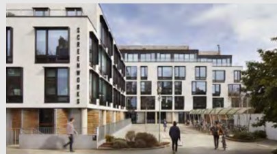
Screenworks Building: £1.6m invested on heatpump installation across 5 floors
