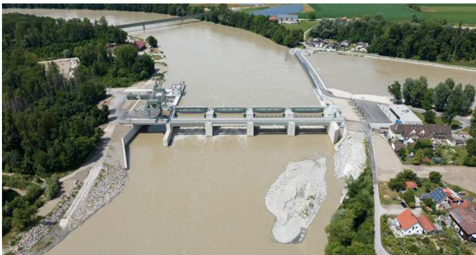
Jettenbach weir: The newly built weir on the Inn River controls the inflow of water to the run-of-river hydropower plant.
