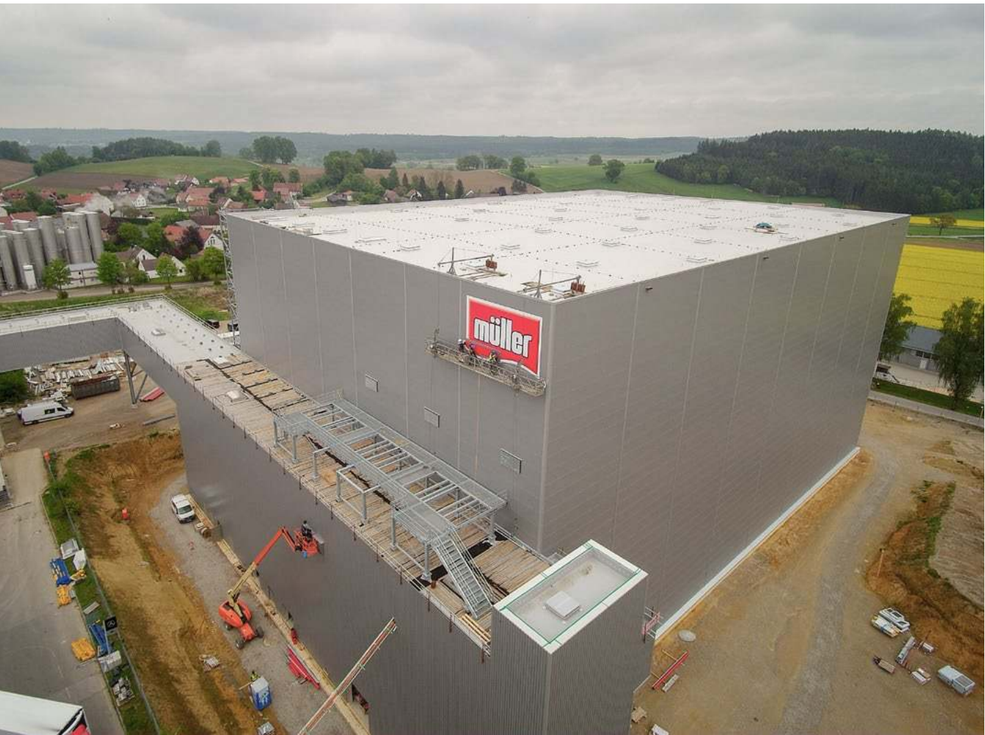
Construction of the high-bay warehouse in Aretsried
