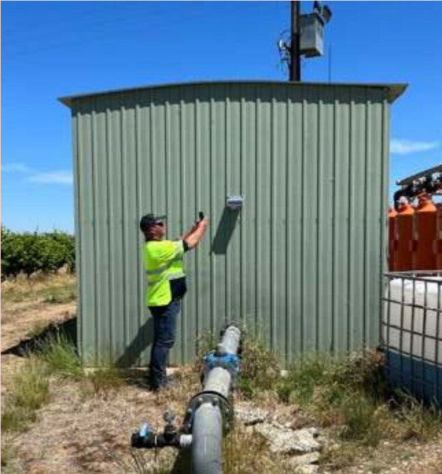
Entering a meter reading into the smart meter online portal to validate a smart meter installation.
