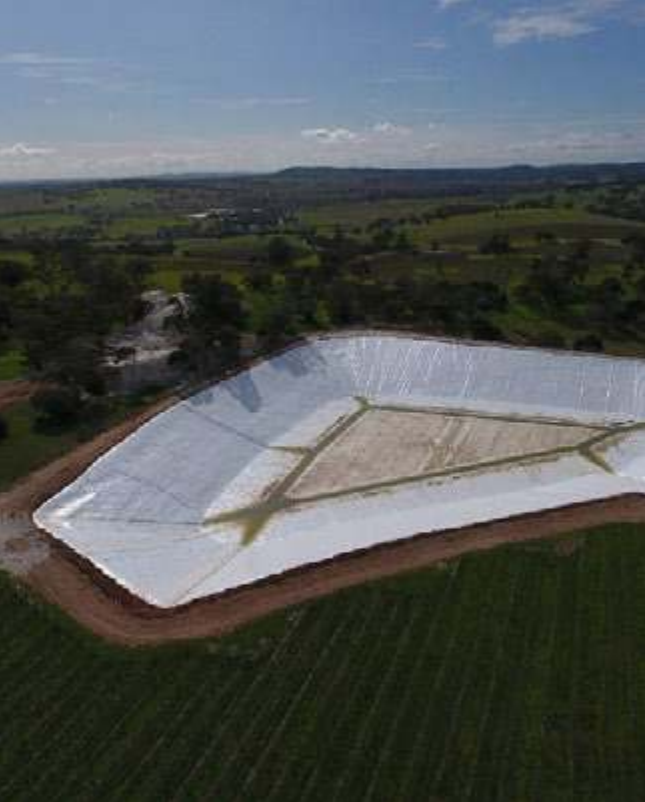
Dam cover replacement and cover installation at Zilm.
