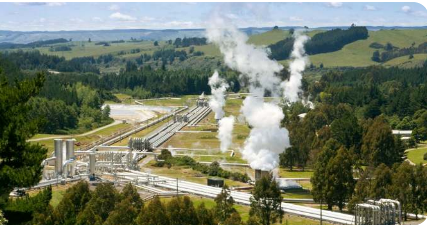
PHOTO: Geothermal production facility.
