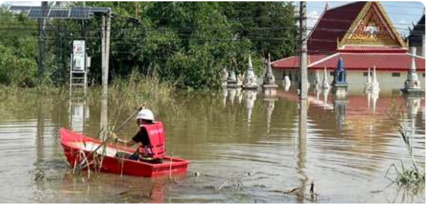
▲ Base station flooding incident caused by extreme weather conditions
