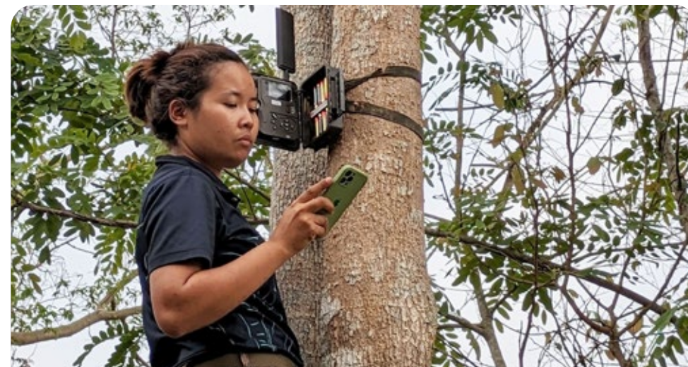
▲ Installation of Elephant Smart Early Warning System
