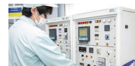
We promote work automation, safety, and efficiency through control panels.
