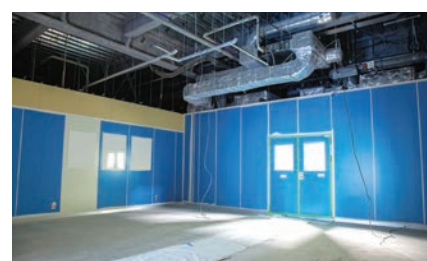
We are in the midst of construction of the CR's expansion. (as of April 2023)
