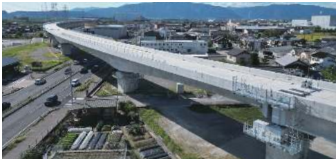
Construction works of the Masada Daisan Viaduct and other 2 bridges (PC Superstructure) on Tokai-Kanijo Expressway
