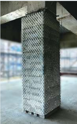
Column fabricated using 3D printing technology
