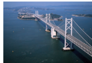
1985 Minami & Kita Bisan-Seto Bridges [substructure, North segment]
