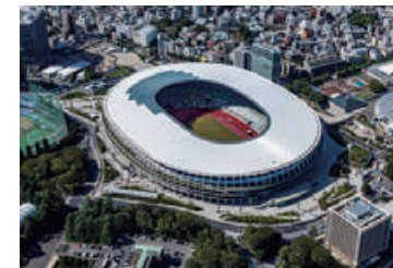
2019 Japan National Stadium
