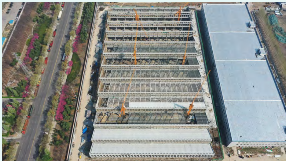
The construction site of smart printing and dyeing upgradation project
