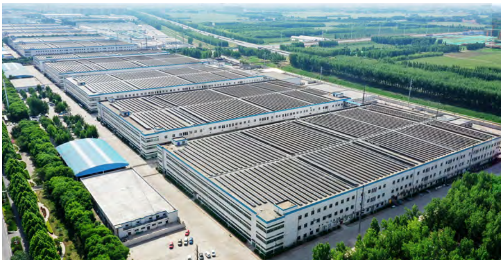
Aerial view of the solar photovoltaic systems on the rooftop of Weiqiao's plants
