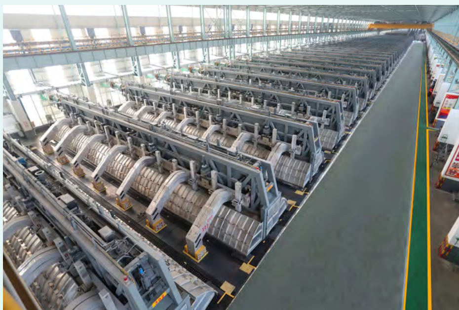
Weiqiao's 600kA super-large anode pre-baked electrolytic cell
