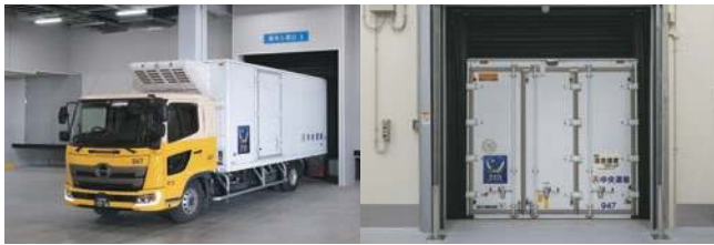
Dock shelters that prevent the intrusion of outside air through the gaps between facility openings and vehicles
