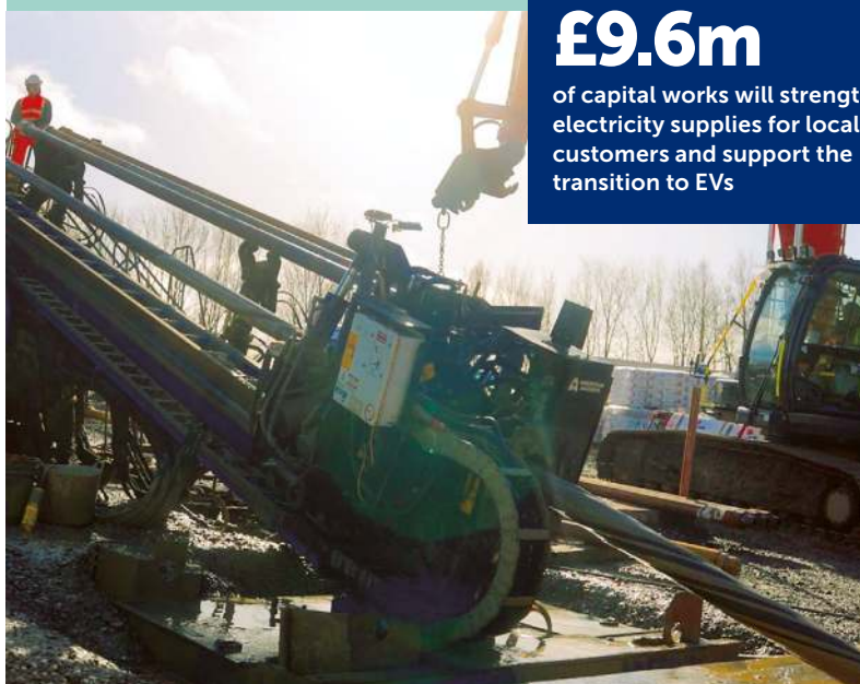
Our underground cables are keeping motorists moving on the M27 motorway
