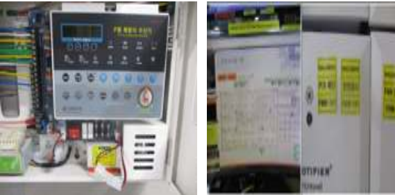
Improving p-type fire sensor receivers – Before (left) and After (right)
