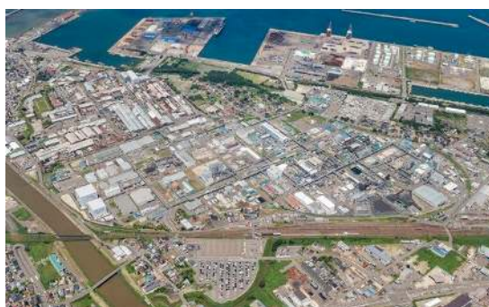
Shin-Etsu Chemical Naoetsu Plant
