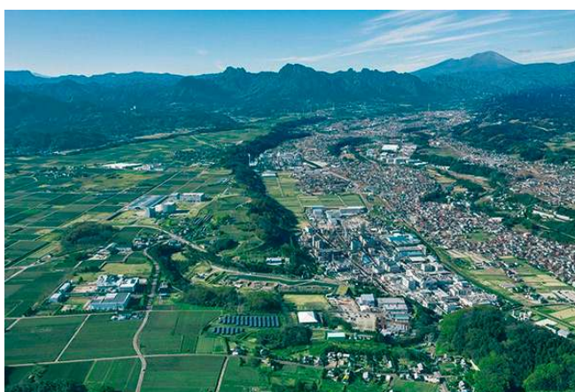
Shin-Etsu Chemical Gunma Complex
