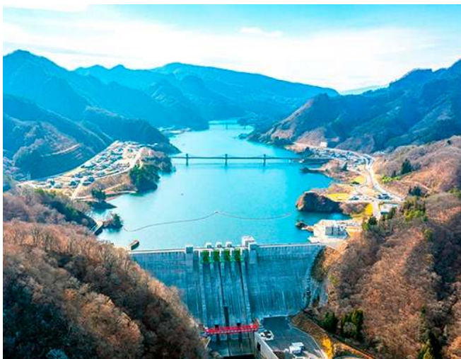
Hydroelectric power plant in Gunma Prefecture
