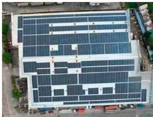
Power generation facilities at Shin-Etsu Magnetics Philippines, Inc.
