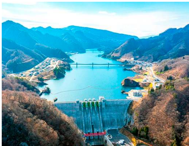
Hydroelectric power plant in Gunma Prefecture
