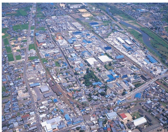
Panoramic view of Takefu Plant
