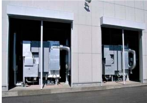
Absorption type refrigerators
