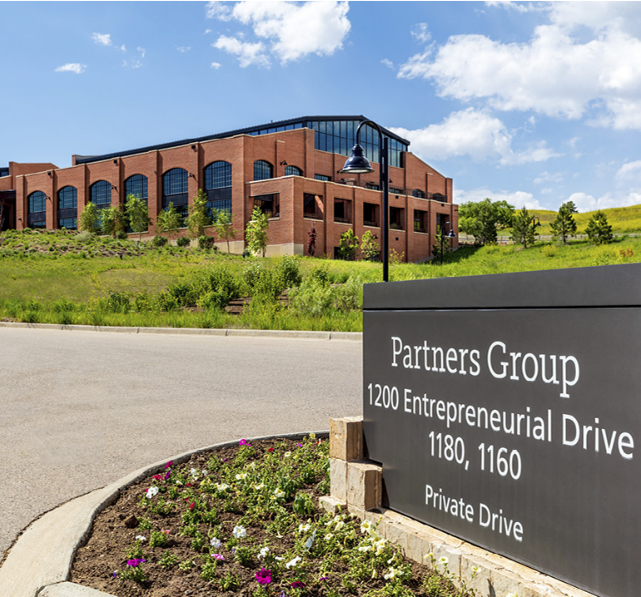
Partners Group campus | Denver, USA
