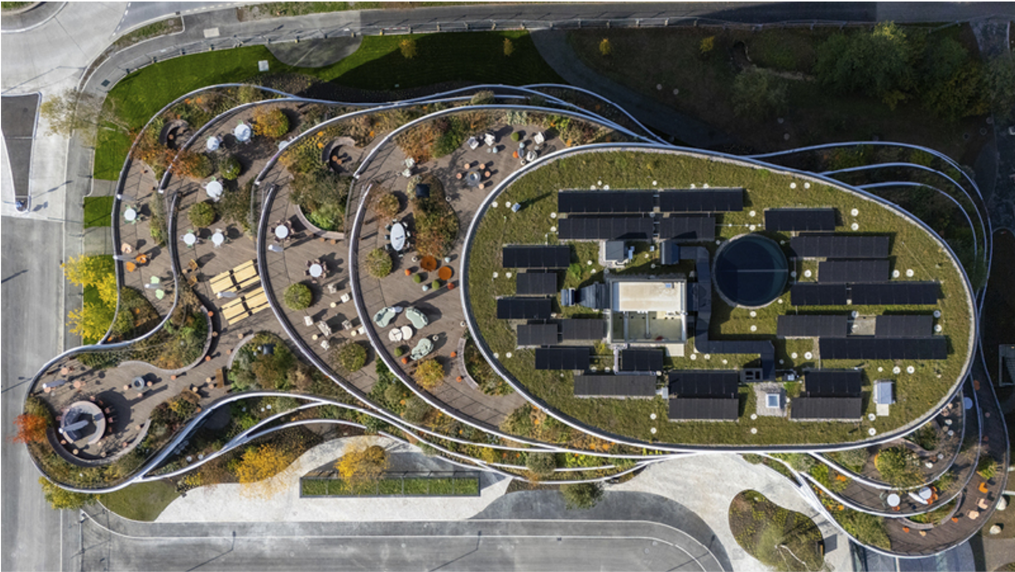
Partners Group campus | Baar-Zug, Switzerland
