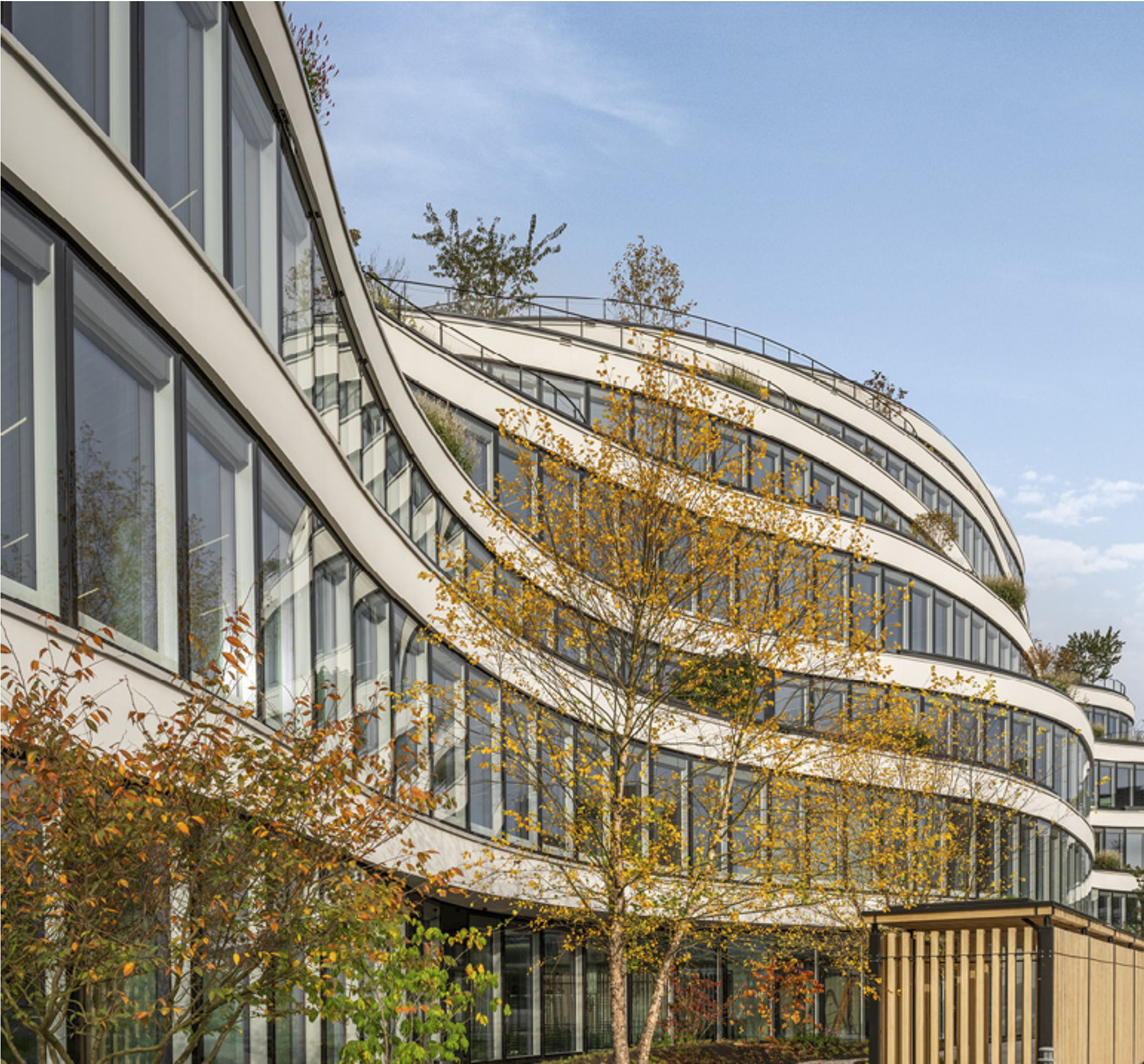
Partners Group campus | Baar-Zug, Switzerland
