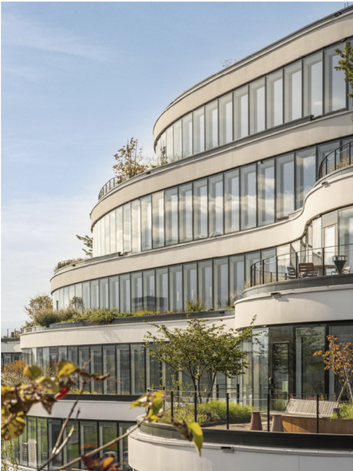
Partners Group campus | Baar-Zug, Switzerland
