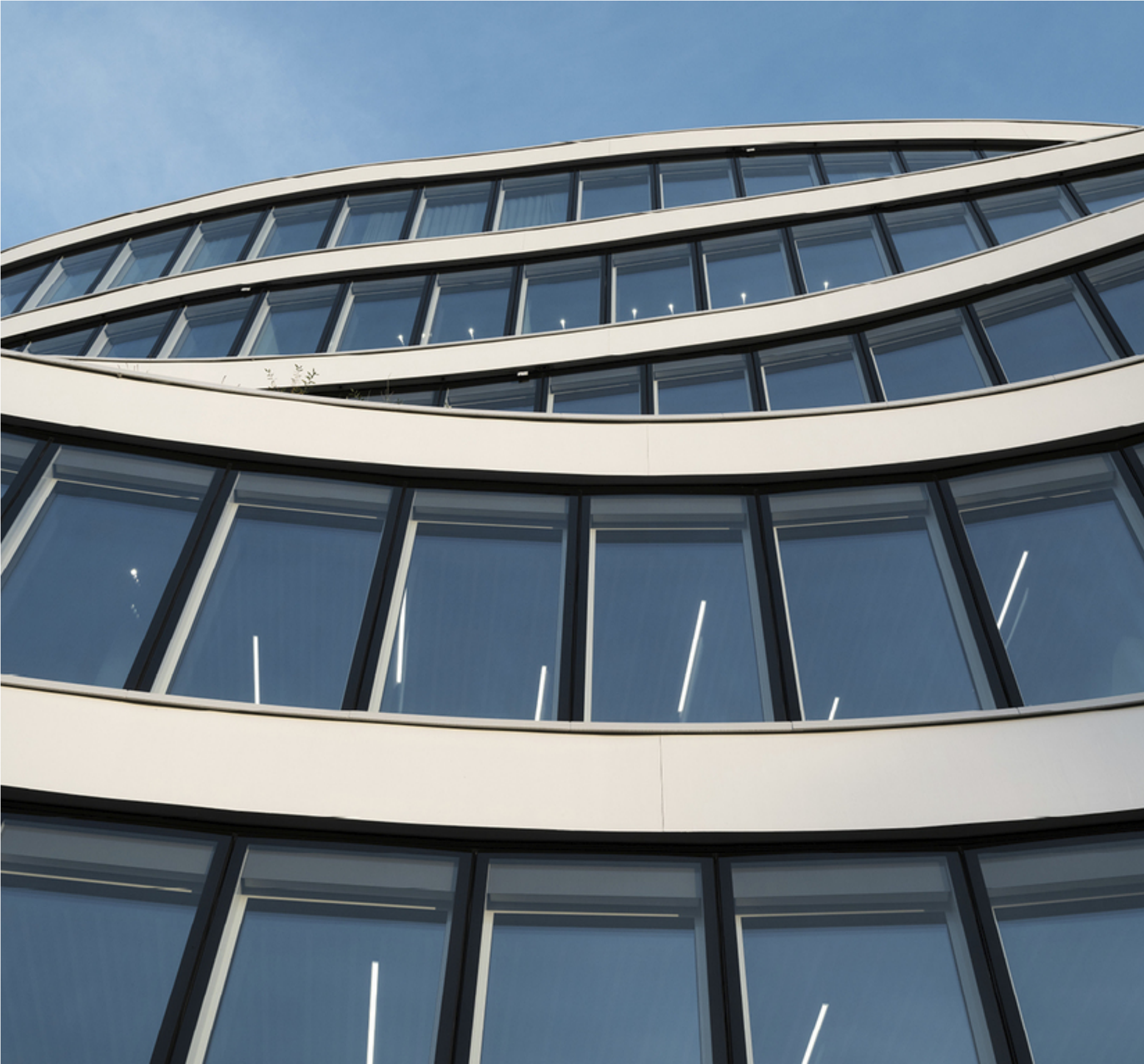
Partners Group campus | Baar-Zug, Switzerland
