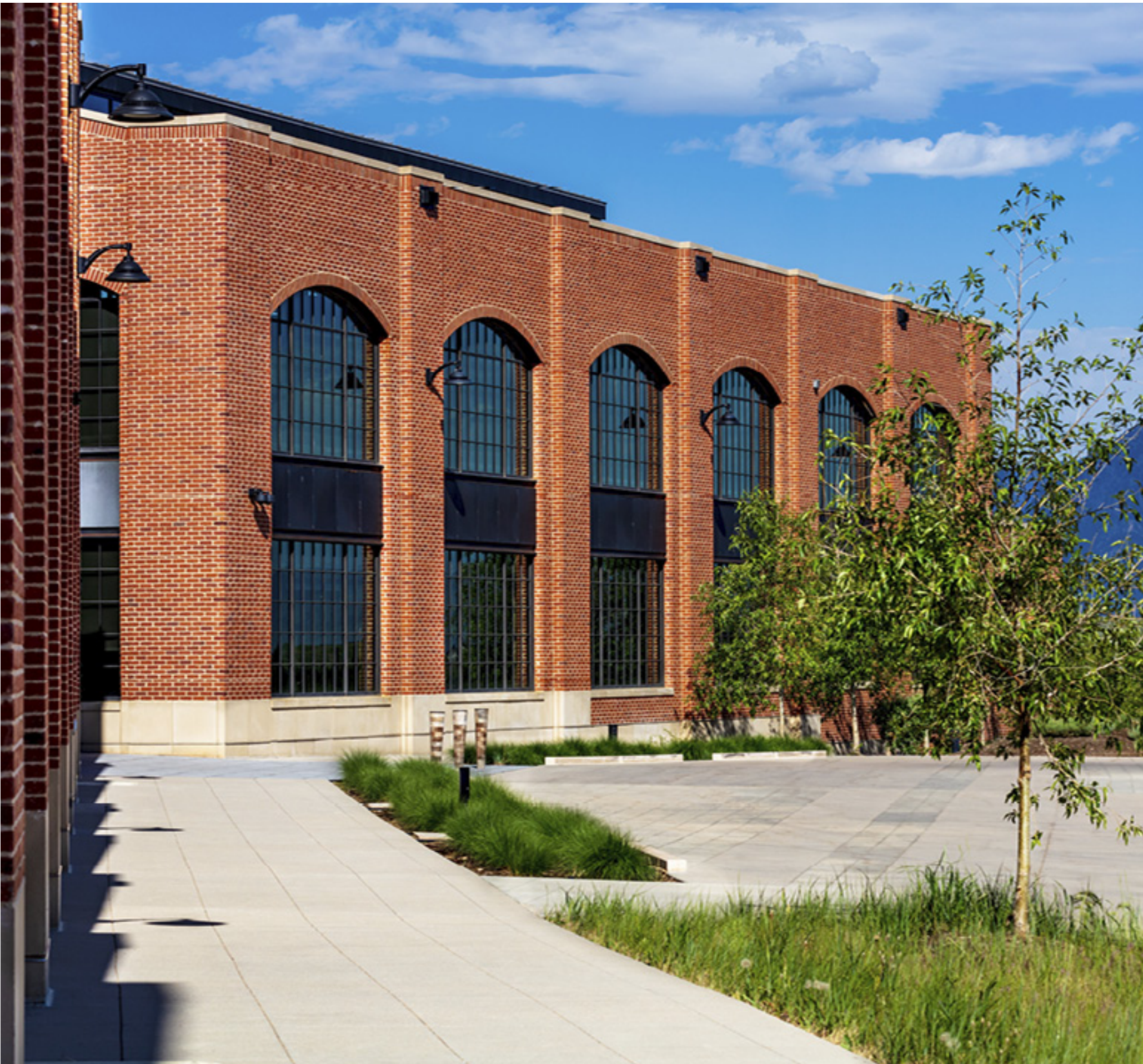
Partners Group campus | Denver, USA
