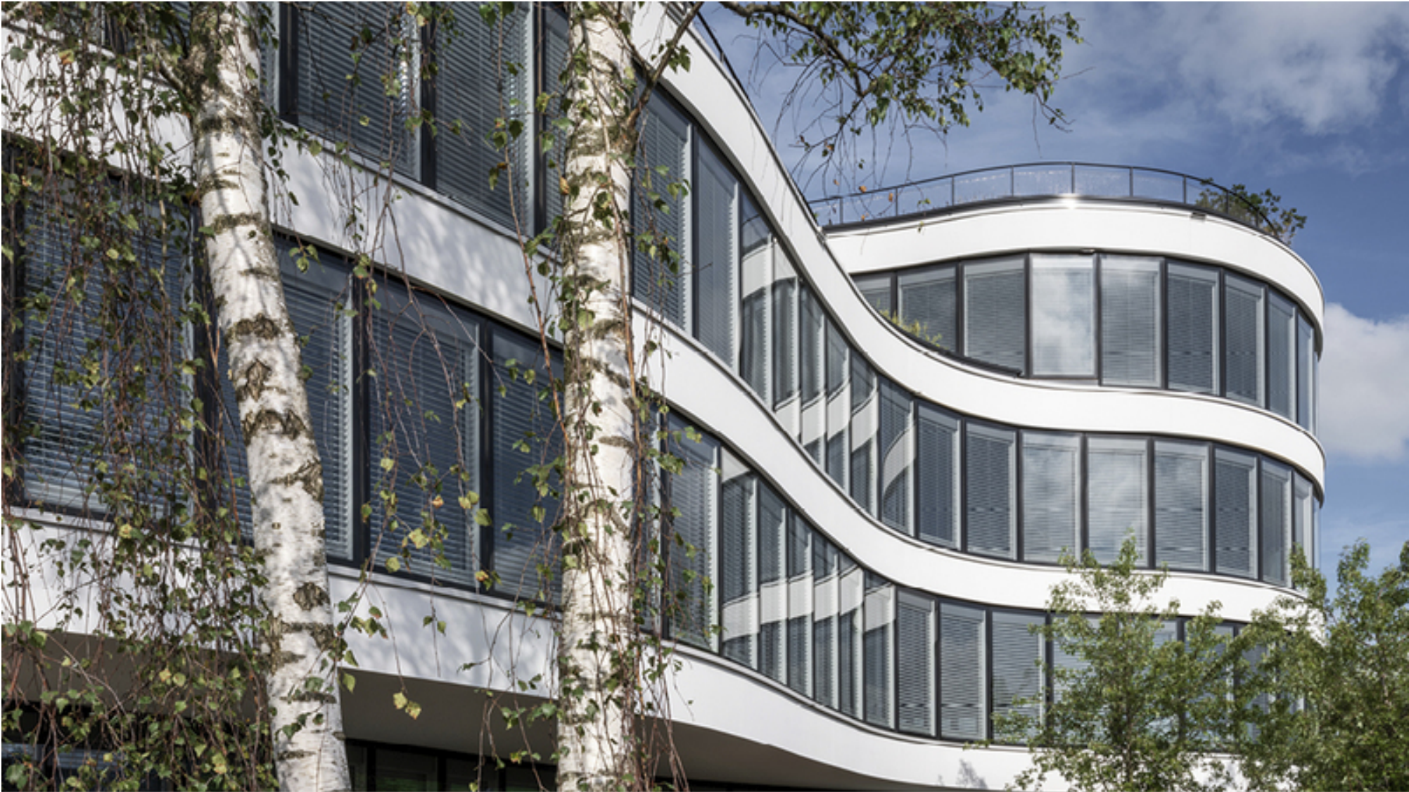
Partners Group campus | Baar-Zug, Switzerland
