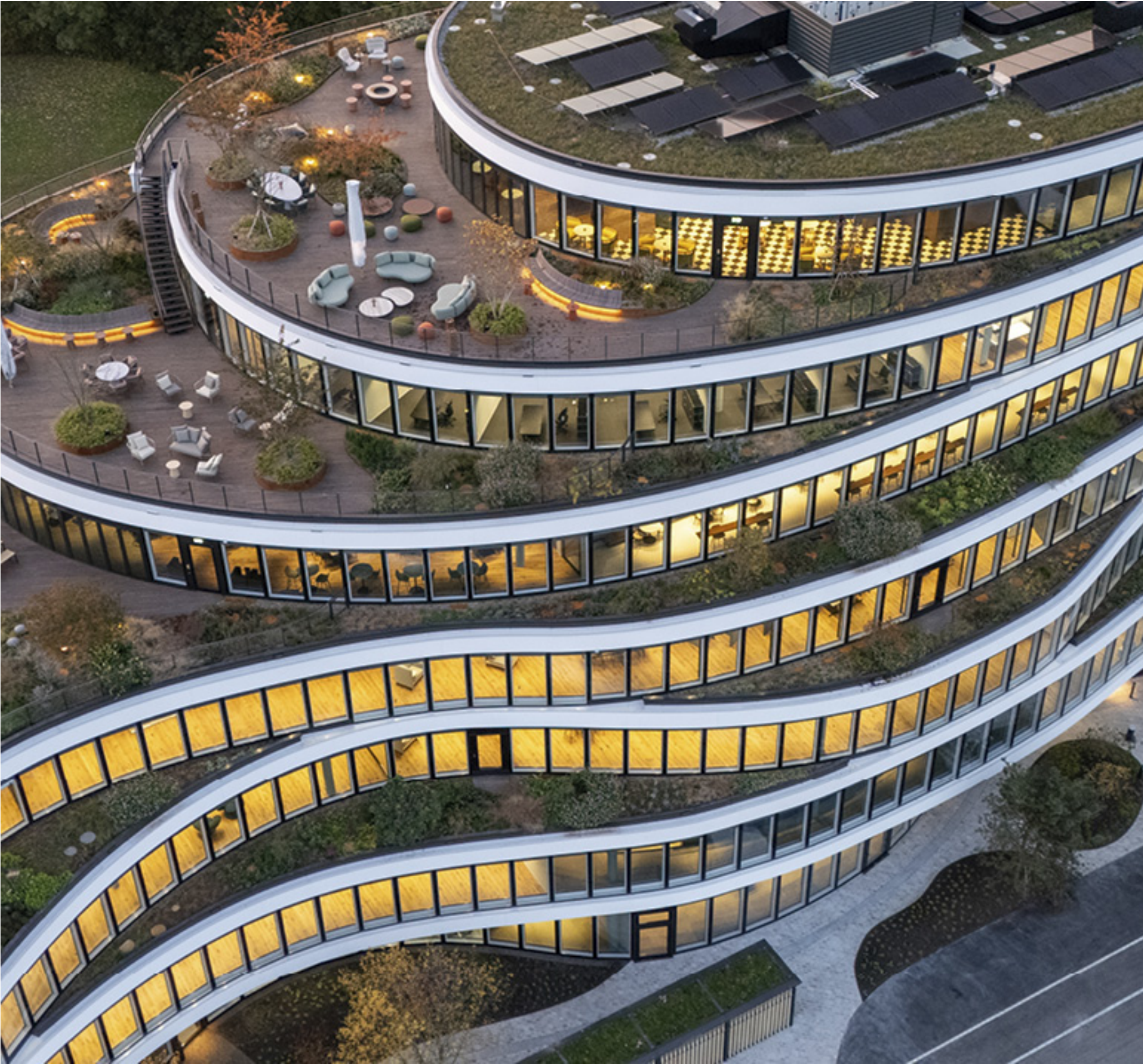
Partners Group campus | Baar-Zug, Switzerland
