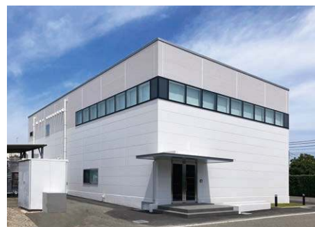
Otsuka Group Energy Management Building
