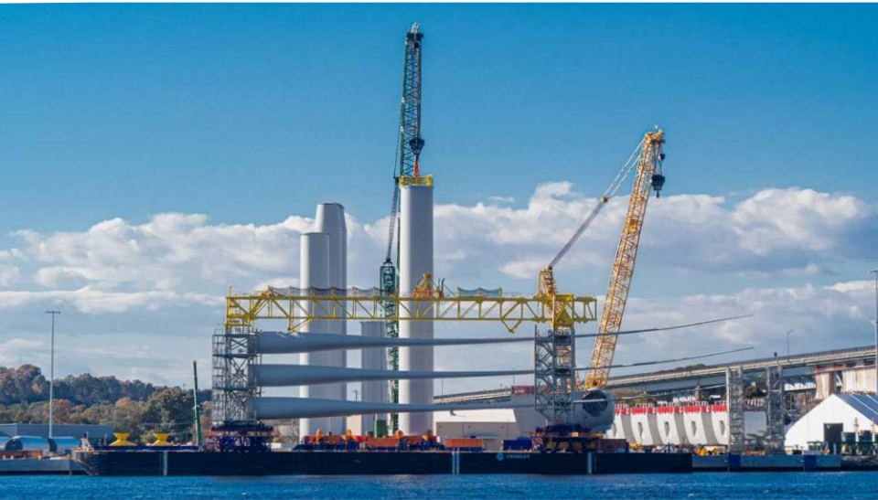
↑ Load-out of blades, South Fork, Connecticut, the US.
