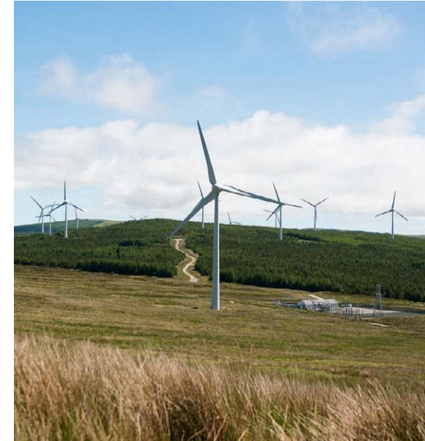
↑ Sorne wind farm, Donegal, Ireland.
