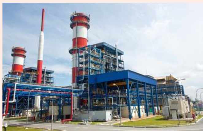
PacificLight Power's existing 830 MW CCGT plant, which will operate in conjunction with the upcoming 670 MW CCGT plant.
