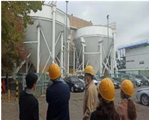
wastewater treatment facility.jpg
