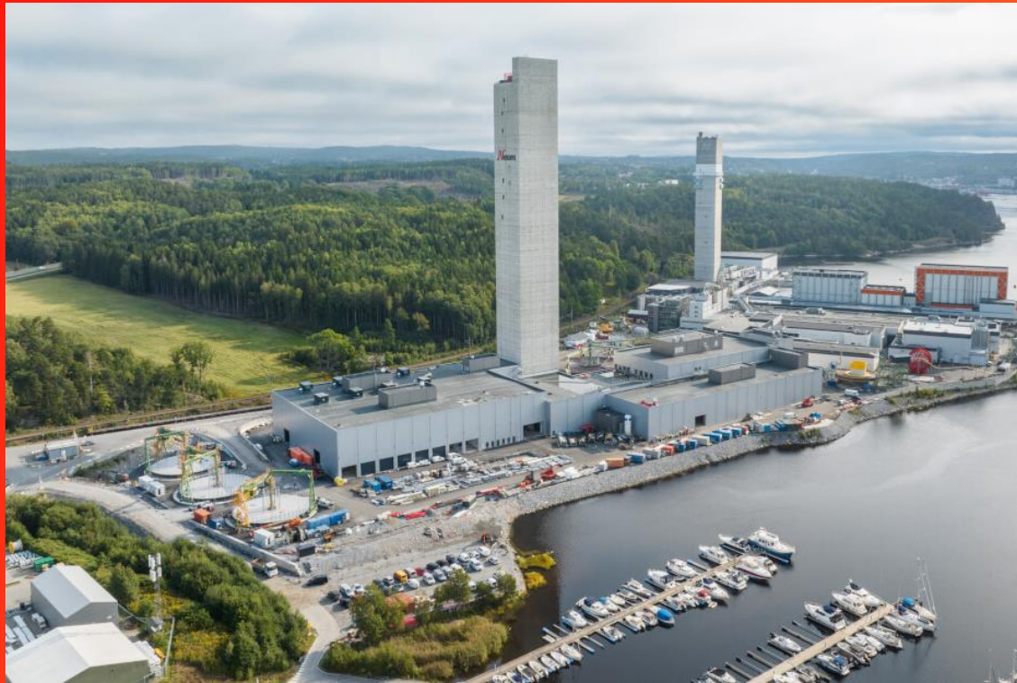
Extension of the Halden plant (Norway)
