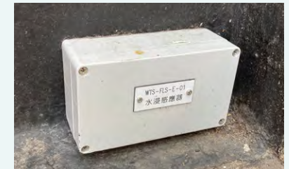
Installation of flooding sensors at station entrances or exits
