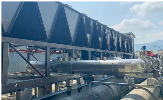
Chiller replacement at Kam Sheung Road Station
