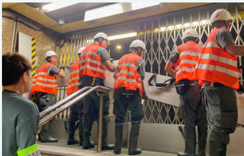
Installation of flood boards at Wong Tai Sin Station
