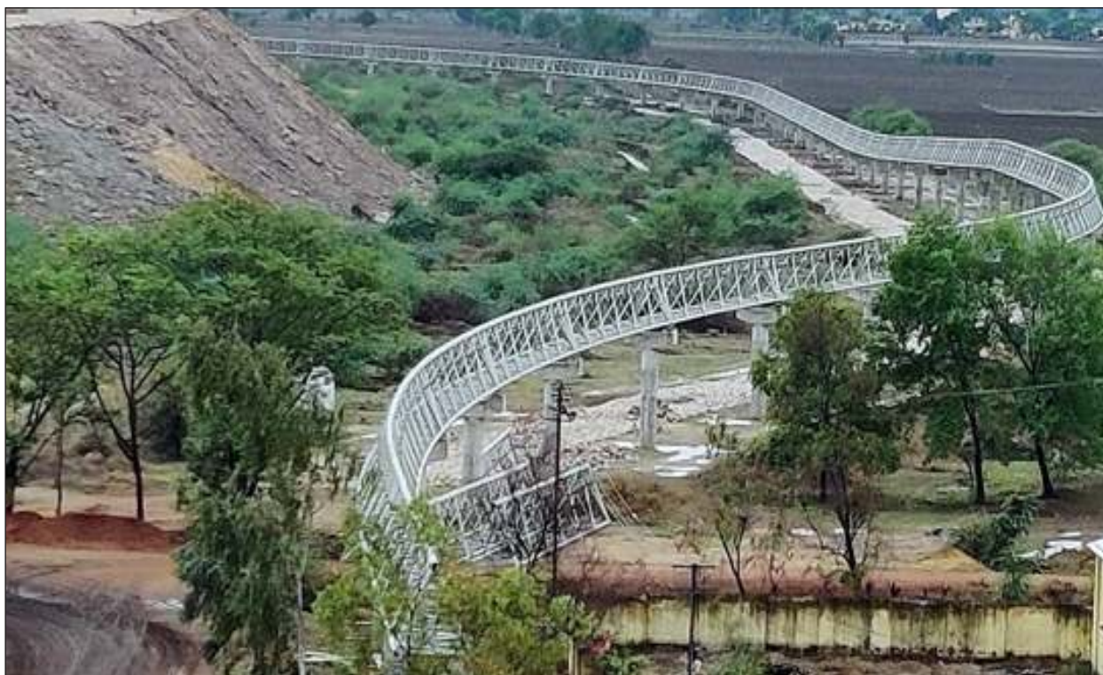
Chandrapur STPS Coal Pipe Conveyor Project PC01
