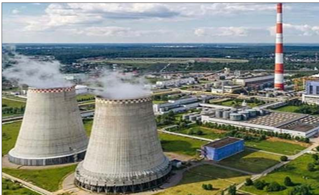
Koradi Thermal Power Station
