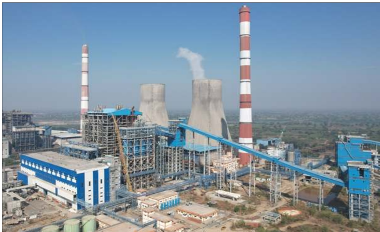
Bhusawal Thermal Power Station
