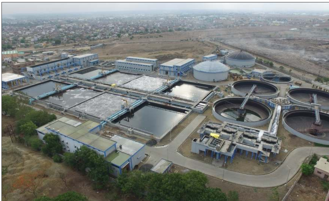
Sewage Water Treatment Plant
