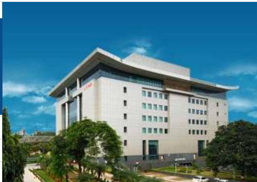
LTM Headquarters, Powai, Mumbai
