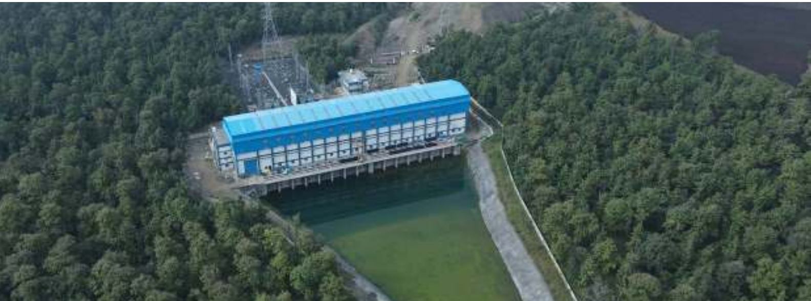
Pump House 3, ISP Parwati Phase I&II Micro Lift Irrigation Scheme, Madhya Pradesh
