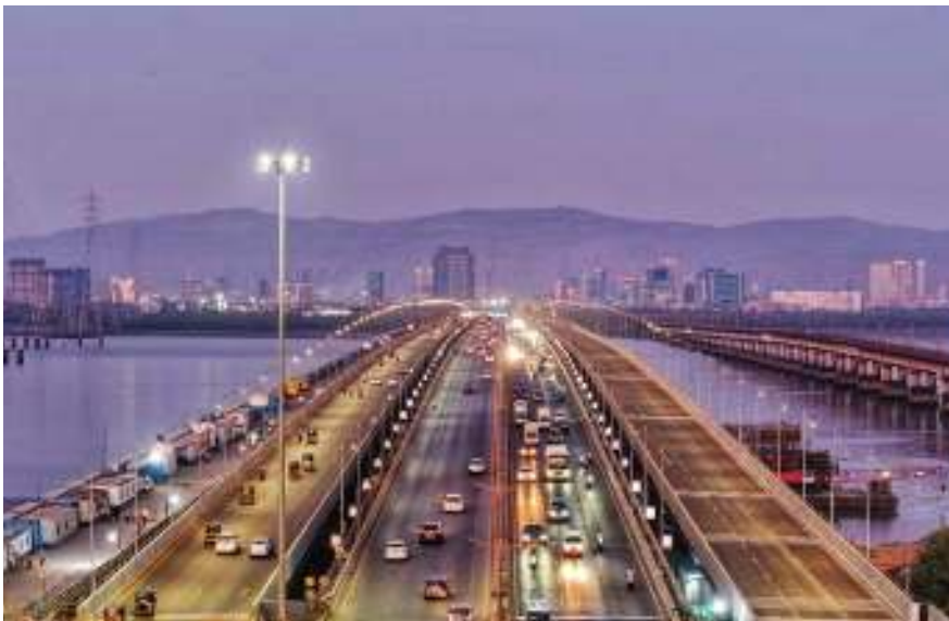
Thane Creek Bridge III - connecting Mumbai & Navi Mumbai, Maharashtra
