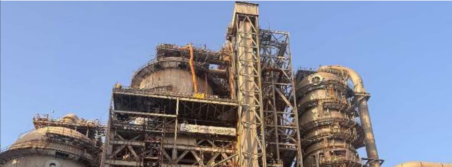
Debottlenecking Project for HOFCC and ECR units, Petro Rabigh, Kingdom of Saudi Arabia
