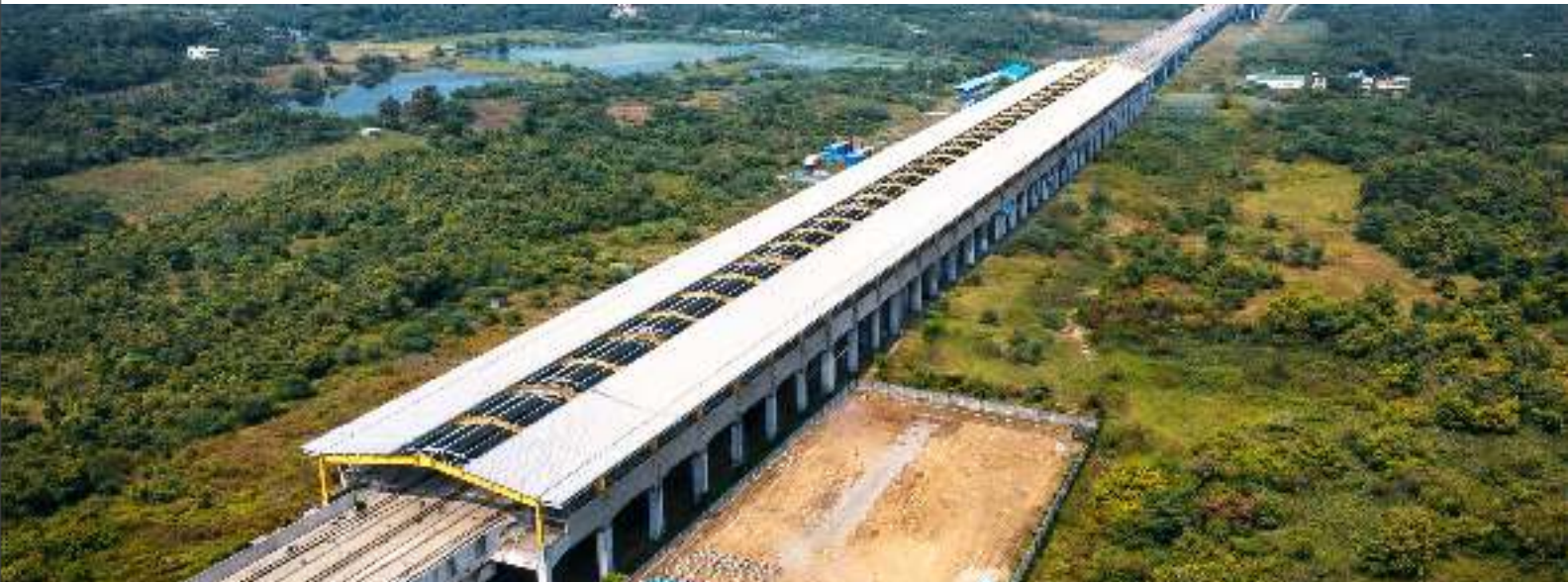
Mumbai-Ahmedabad High-Speed Rail (MAHSR) Project, Bilimora Station in Gujarat
