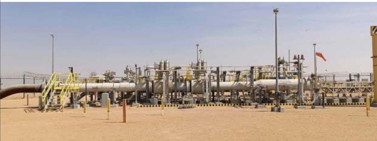
Jafurah Export Pipeline Project for Saudi Aramco, Kingdom of Saudi Arabia
