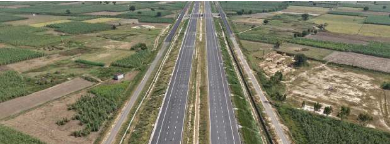
Ganga Expressway (MGEP), connecting Meerut to Prayagraj, Uttar Pradesh
