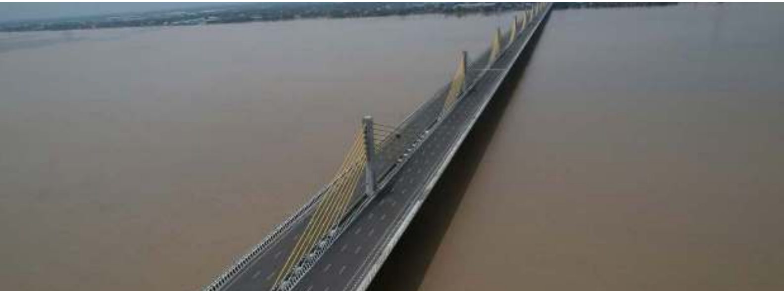
Kachchi Dargah Bridge Project (over the Ganges), Bihar
