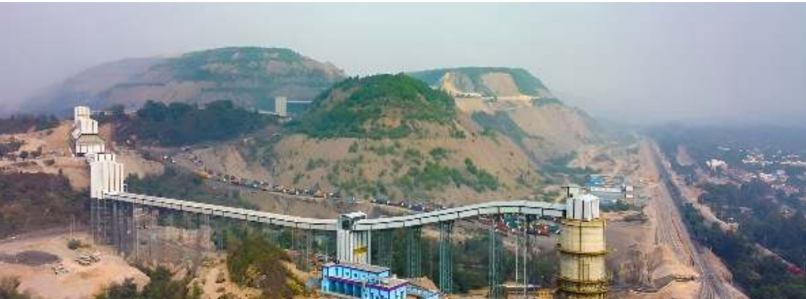
Coal Processing and Load-Out Package at the Dudhichua Mines, Madhya Pradesh
