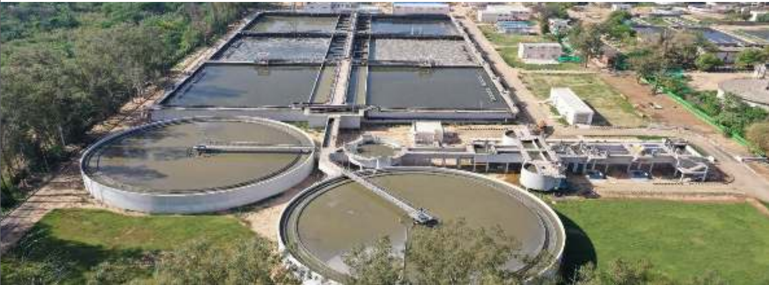
136 MLD Sewage Treatment Plant, Diggian, Chandigarh
