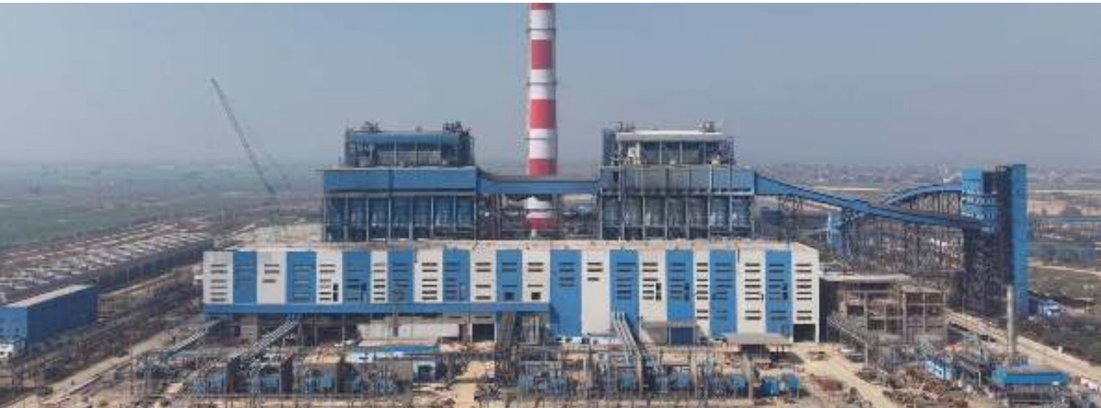
2x660 MW Buxar Thermal Power Plant, Bihar
