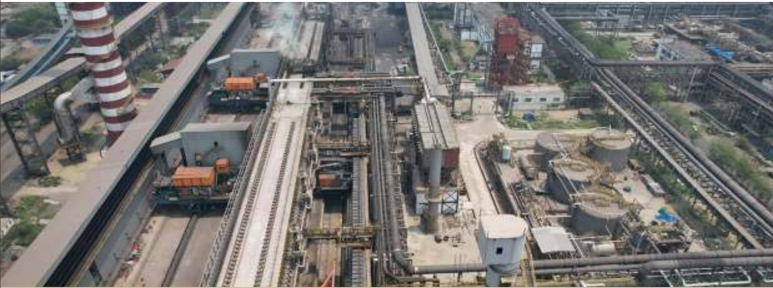
Kalinganagar Coke Oven Battery Project, Odisha
