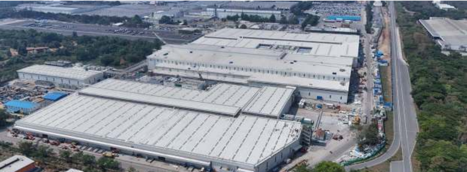
State-of-the-art plant for Toyota Kirloskar near Bengaluru, Karnataka
