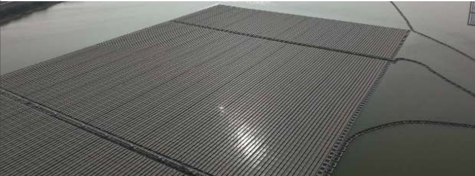
56 MW Floating PV Project, Ramagundam, Telangana
