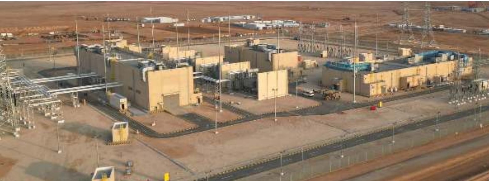
Al Ghat Wind 380/132 kV Bulk Supply Point (BSP) # 9084, a critical infrastructure project supporting a 600 MW onshore wind power plant in the Riyadh province of Kingdom of Saudi Arabia
