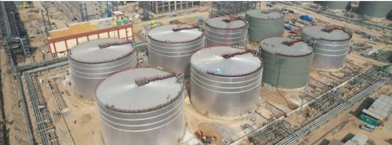
Offsite Tankages and Bullets (incl. all associated facilities) for Indian Oil Adani Ventures Limited (IAVL) at IOCL Panipat Refinery, Haryana
