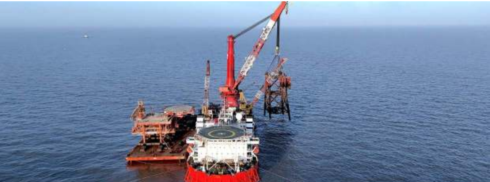
India's First Decommissioning Project - Tapti Facilities Decommissioning, British Gas Exploration & Production India Limited (BGEIPL)
