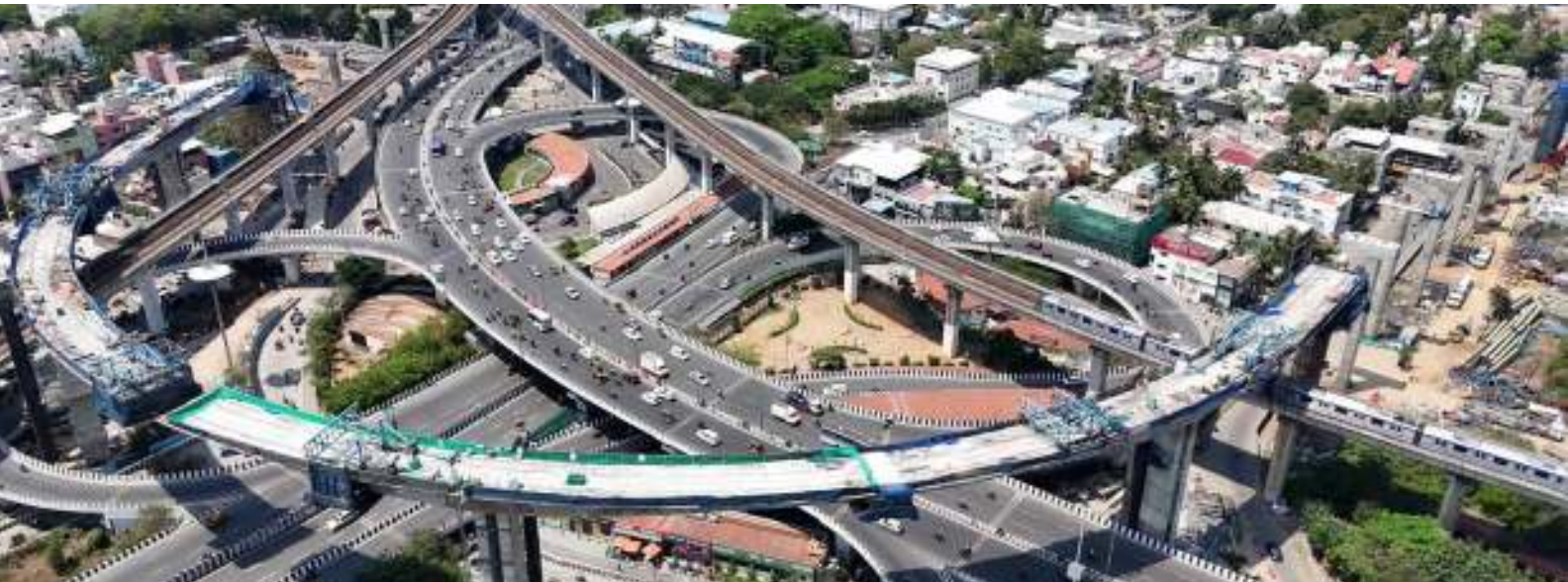
The sharpest curve at a 125m radius at the Kathipara Junction, Chennai Metro Rail Phase 2, Tamil Nadu
