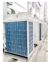
New air conditioner external unit
