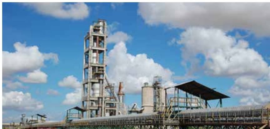
JK White Cement Plant, Gotan
