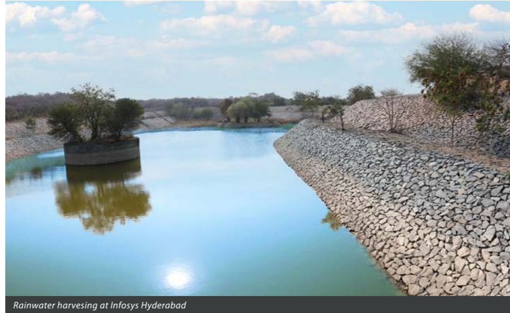
Rainwater harvesting at Infosys Hyderabad
