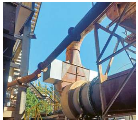
WASTE HEAT RECOVERY
