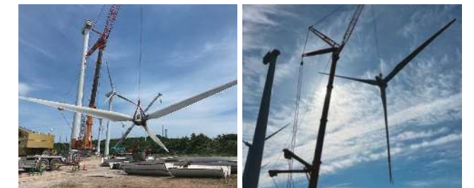
Dismantling wind turbines
