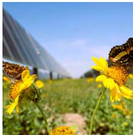
Page 15 Orange Grove Solar is a 130-MW renewable energy facility in operation near Corpus Christi, TX.
