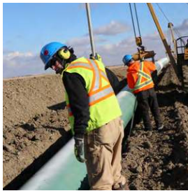
Page 45 Construction activities in western Canada on our LP Mainline.
