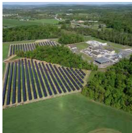
Page 21 Heidlersburg Solar is a 2.5 MW solar project which offsets some of the power consumed by GTM's Heidlersburg Compressor Station, along our Texas Eastern gas transmission pipeline.
