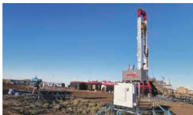
Drilling rig for new wells drilling
