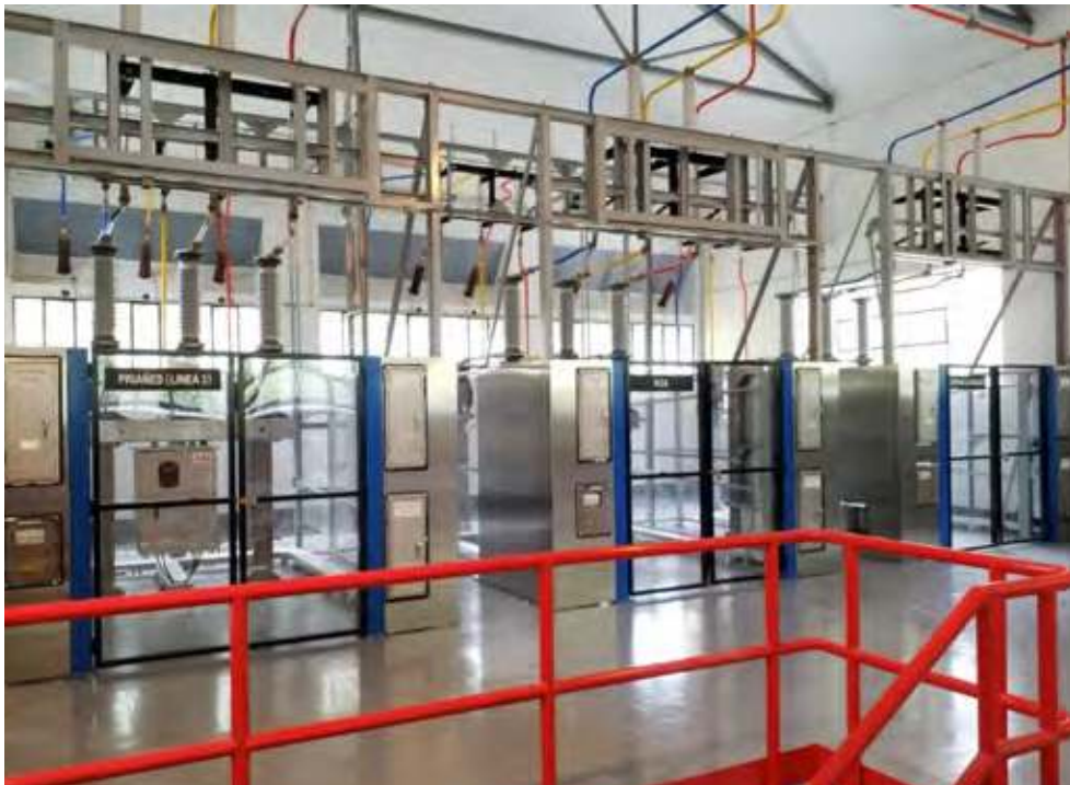
View of the finished works
