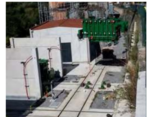
Installation of the new transformor
