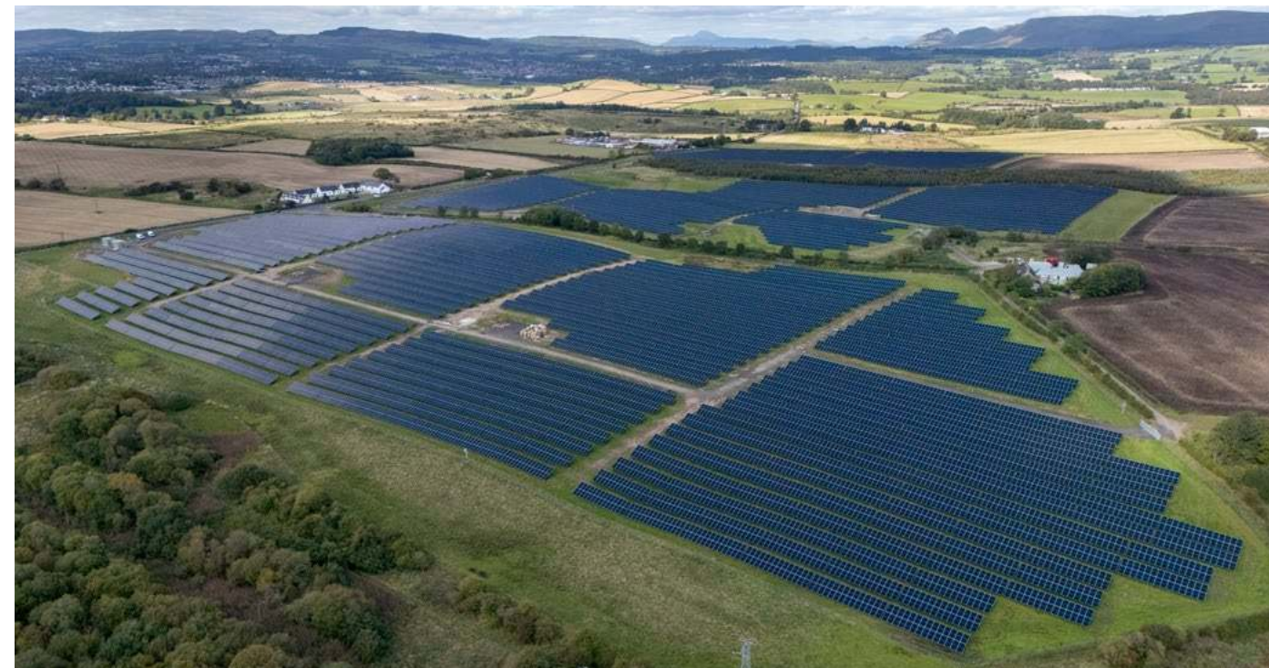
Lochfauld Solar Park
