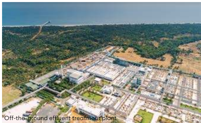
Off-the-ground effluent treatment plant
