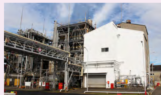
New dissolution and separation recycling facility
