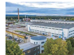
Fürstenwalde Production Plant, Germany
