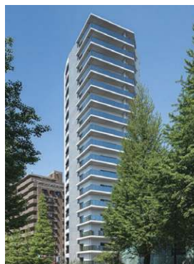
Rebuilding business PREMIST Shirokane
