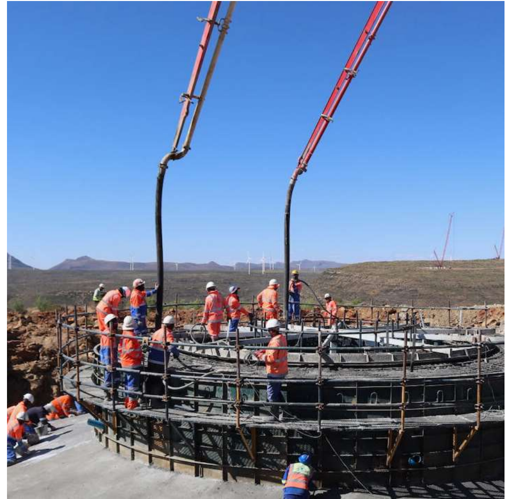
Koruson 2 wind and solar project under construction in South Africa, June 2024
