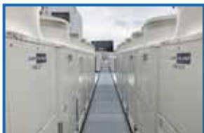
Upgrading of air-conditioning equipment (Daiwa Ginza)
