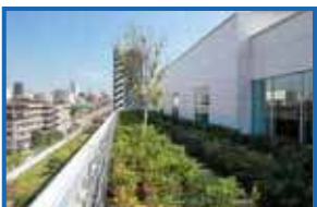
Installation of rooftop garden (Daiwa Azabu Terrace)
