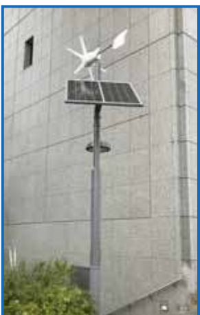
Installation of Solar-Wind Streetlights (Daiwa River Gate)
