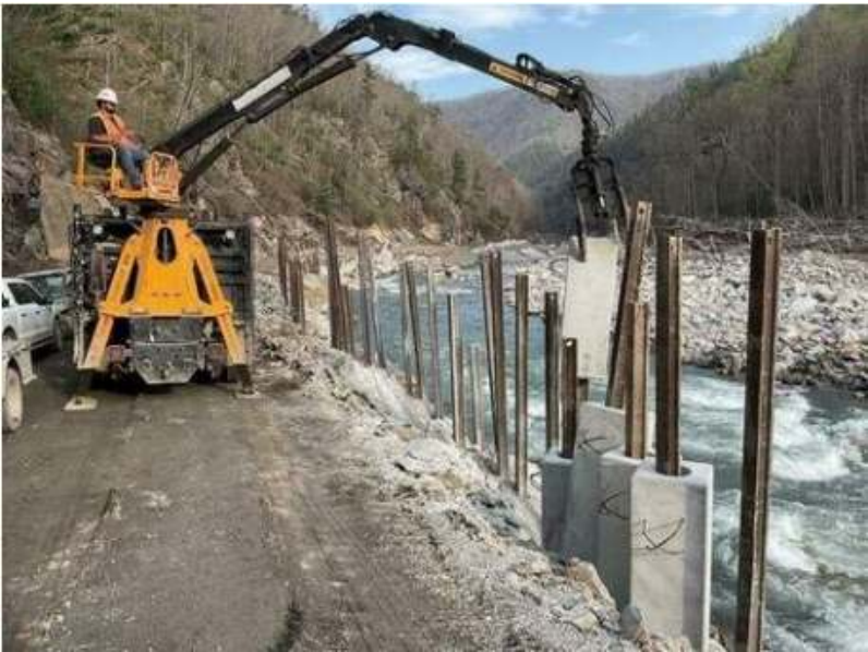
During reconstruction of the Blue Ridge Subdivision following Hurricane Helene, sections of track recovered from the river were repurposed to reinforce the rail bed with rail-pile retaining walls. This innovative approach reduced waste, conserved construction materials, and enhanced infrastructure resilience, demonstrating how recovery efforts can create long-term operational and environmental benefits.
