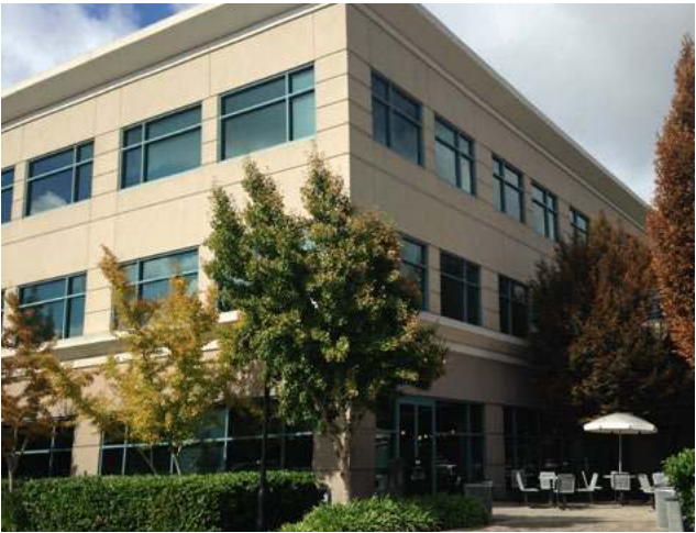
Installed Window Film Reduces Energy Costs, San Jose, California
