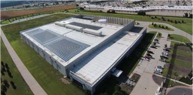
Solar Project at Cisco Data Center, Allen Texas
