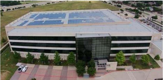
Solar Project at Cisco Data Center, Richardson Texas
