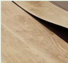
Overlay Flooring Renovation
