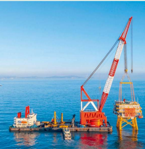
Hoisting of CR Power's "Cangnan No. 1" offshore booster station
