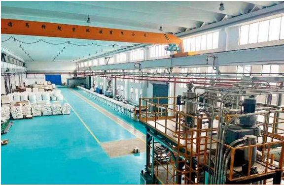
CR Chemical Materials' PET foam production line
