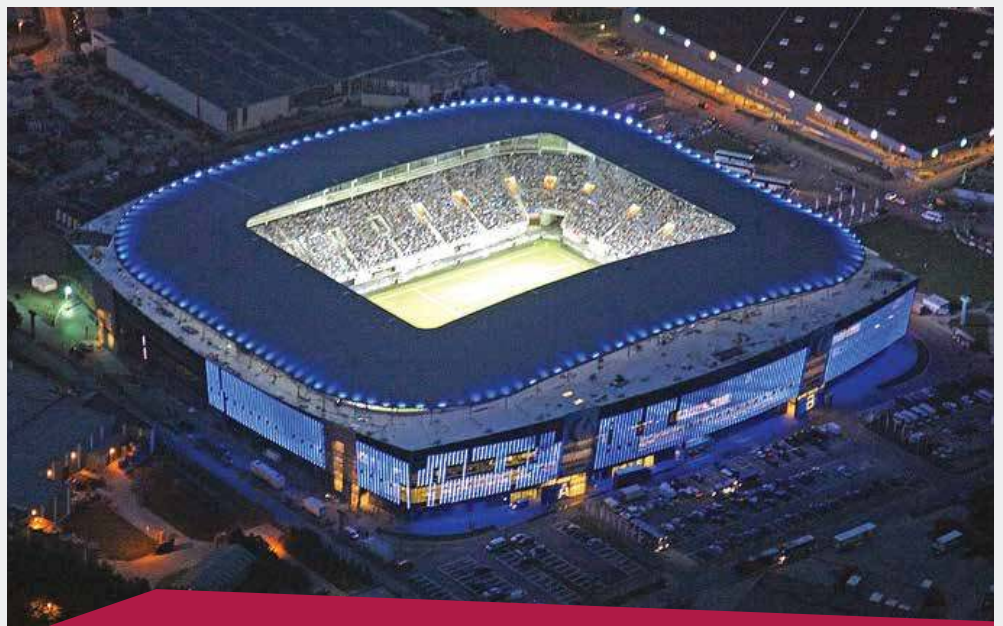
Ghelamco Arena in Ghent, Belgium was designed to be the first ecological stadium in the Benelux and is also an important focus for economic and social regeneration in the urban area. CRH Subsidiaries Ergon and Prefaco produced 18,000 m 3 of structural concrete for the project and provided the design, fabrication and delivery of the concrete elements for the stadium, which was completed in May 2013 and has a capacity for 20,000 supporters.
