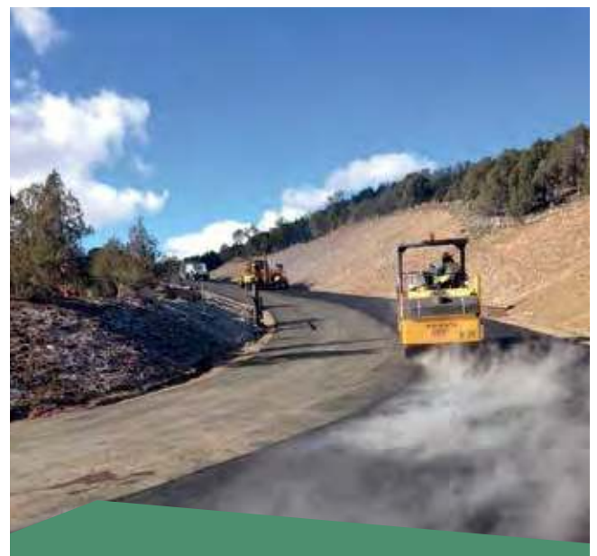
Four Corners Materials, an Oldcastle Materials subsidiary, installed a paved haul road at its Animas Glacier Pit in Colorado, US to reduce dust emissions from the movement of plant and equipment on-site.
