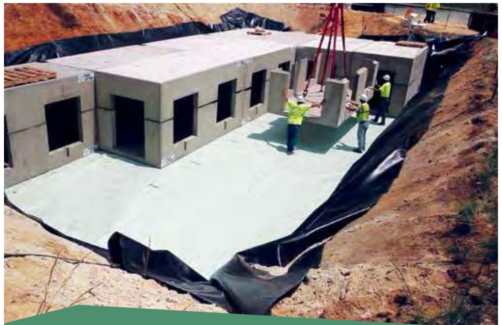
The Storm Capture Total Stormwater Management System produced by Oldcastle Precast, US, shown here being installed at a building site in Triangle, Virginia, offers many solutions for stormwater management needs. The system also assists with control of runoff, preventing storm drain overloading and other downstream issues such as flooding and erosion.
