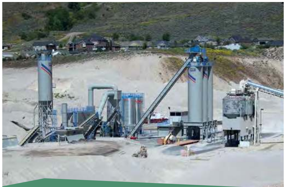
Staker Parson, an Oldcastle Materials subsidiary, has invested in a new asphalt plant at its Brigham North location in Utah, US. The new energy-efficient plant enables the production of warm-mix asphalt and the increased use of recycled asphalt pavement.
