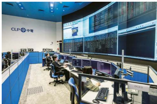
CLP Power's System Control Centre, which marked its 40 th anniversary in 2025, has been operating round the clock to monitor the power system, ensuring a stable and secure electricity supply.
