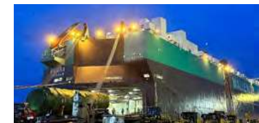
Site for unloading battery factory equipment
