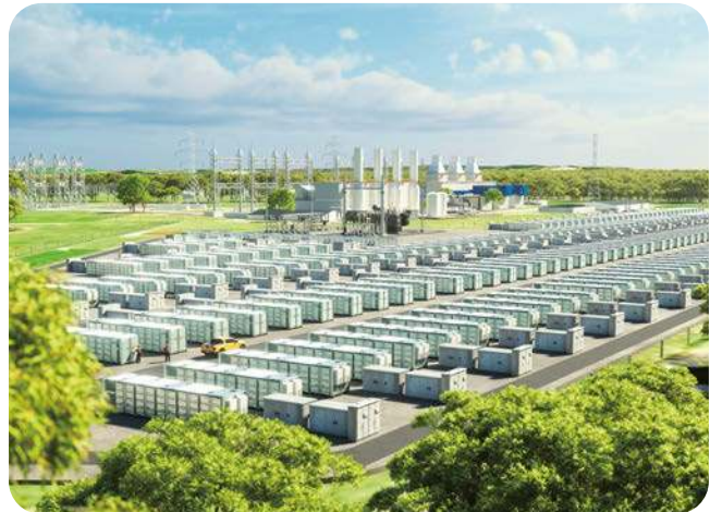
■ EnergyAustralia invests in flexible capacity initiatives such as the Wooreen battery energy storage system in Victoria to support Australia's clean energy transition.
