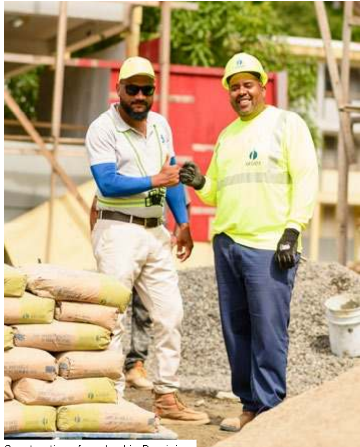
Construction of a school in Dominica
