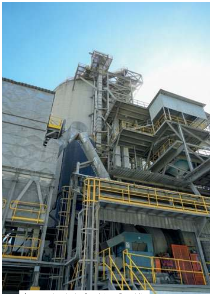
Cement plant in the Dominican Republic
