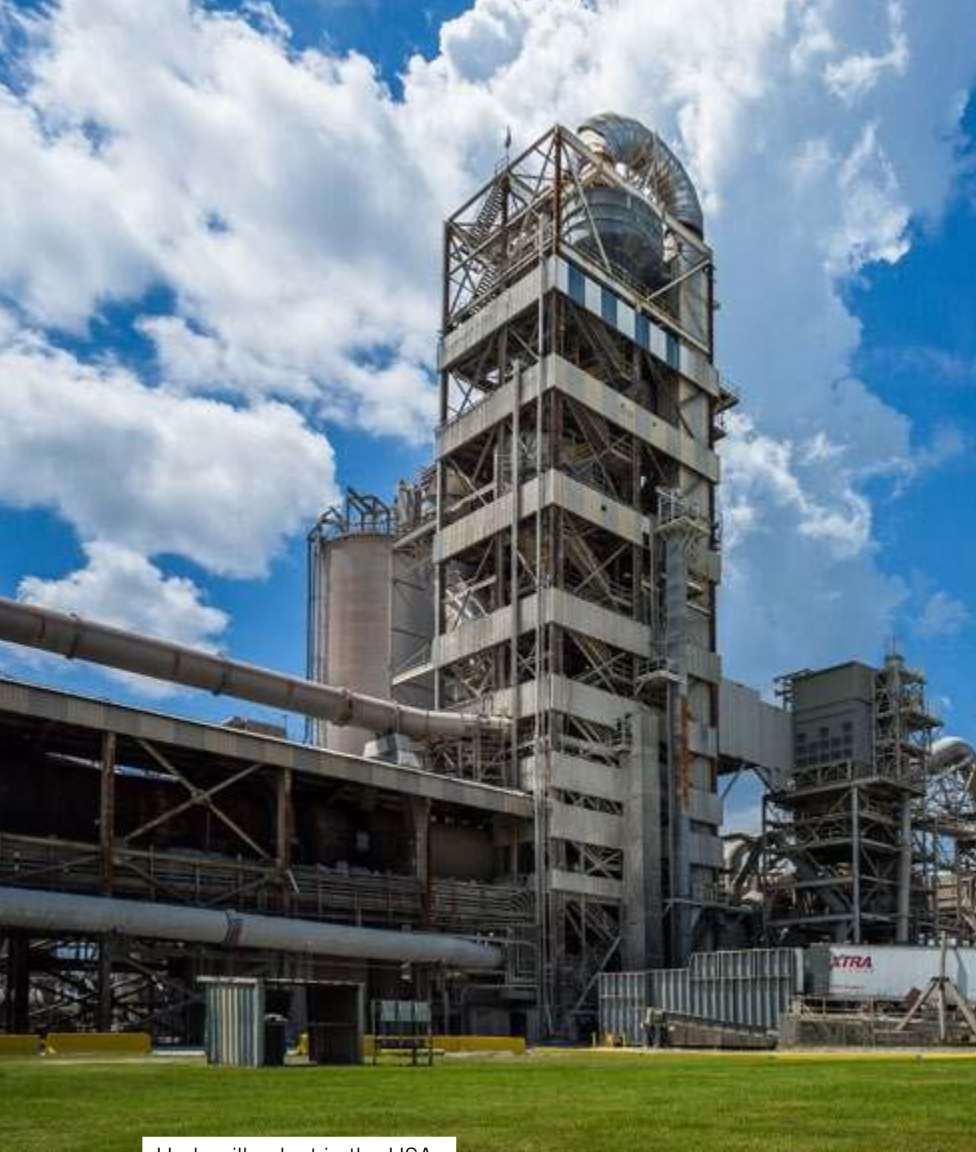
Harleyville plant in the USA.
