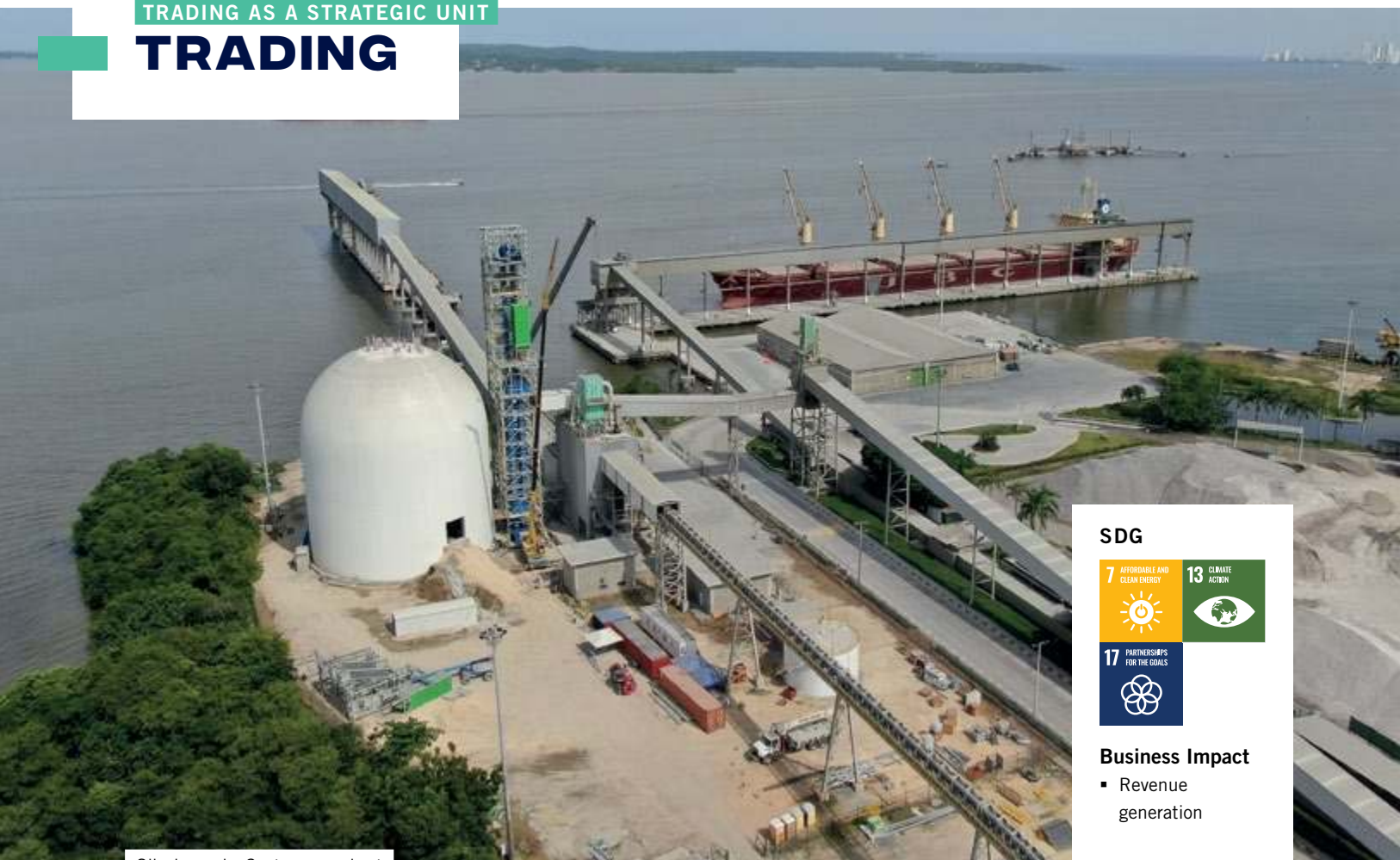
Silodome in Cartagena plant
