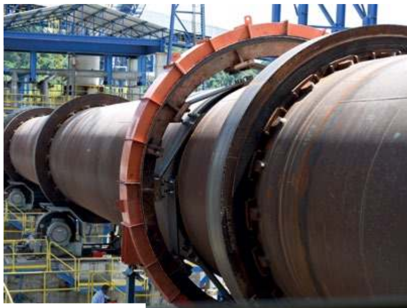
Rioclaro plant in Colombia
