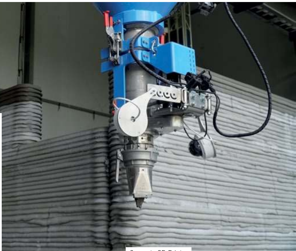
Concrete 3D Printer
