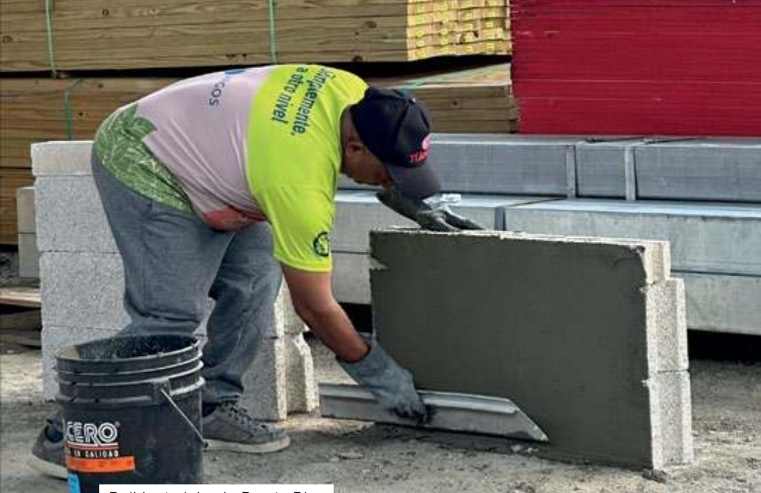
Builder training in Puerto Rico
